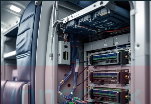
Limited Space and Challenging Cable Routing
